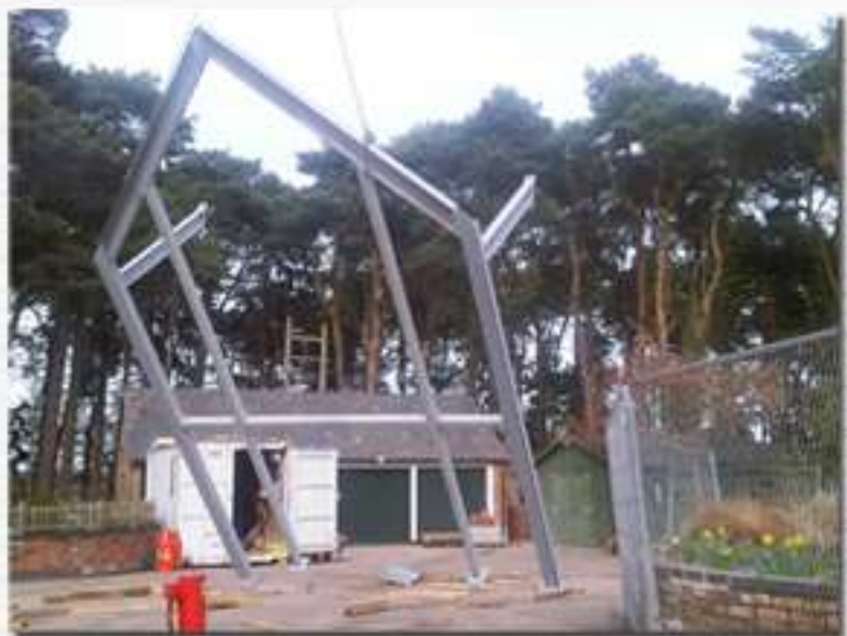
Swimming Pool Steelwork 2
