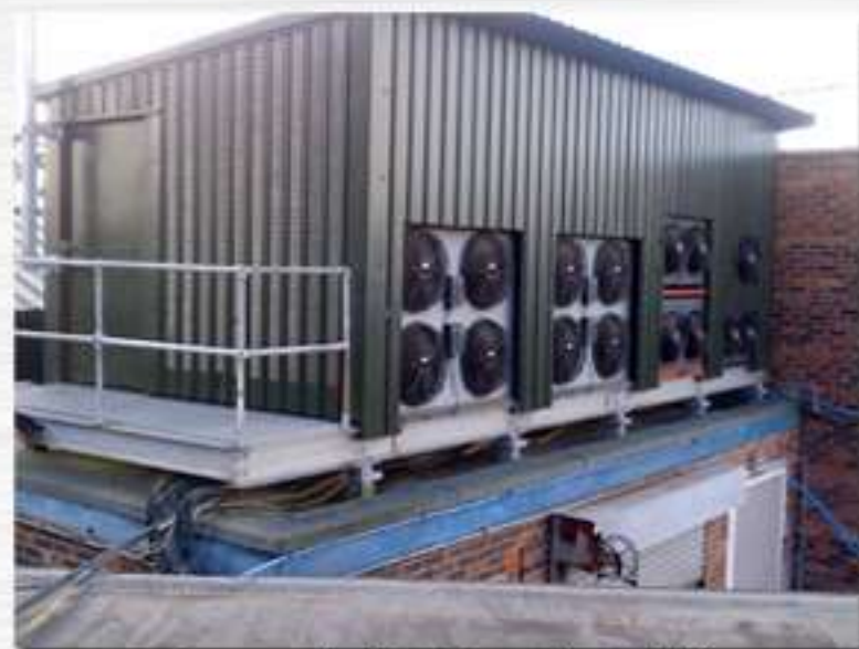
Suspended Refrigeration Building
