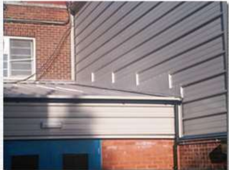
Re-clad and tie in to existing building
