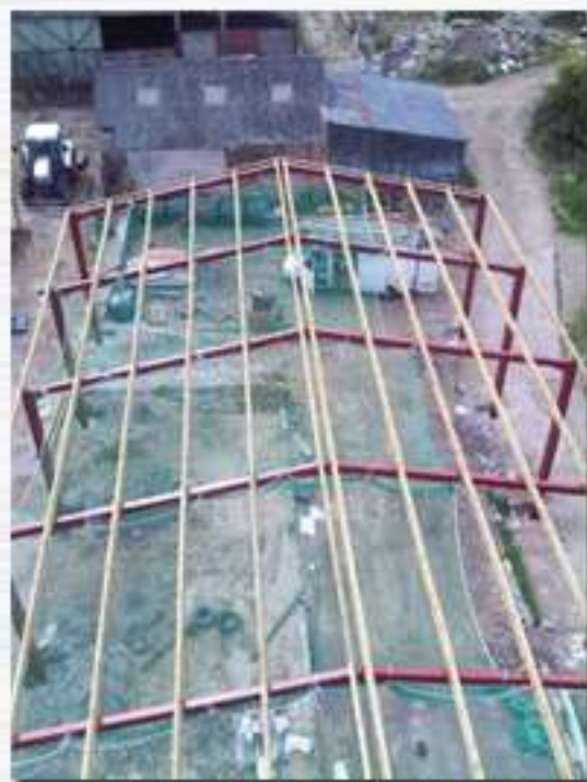
Storage Barn Frame
