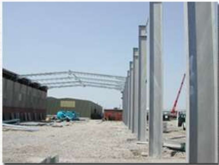
Ercting Steel Frame
