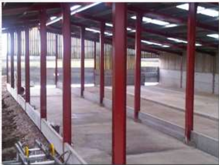
Cowshed in Progress
