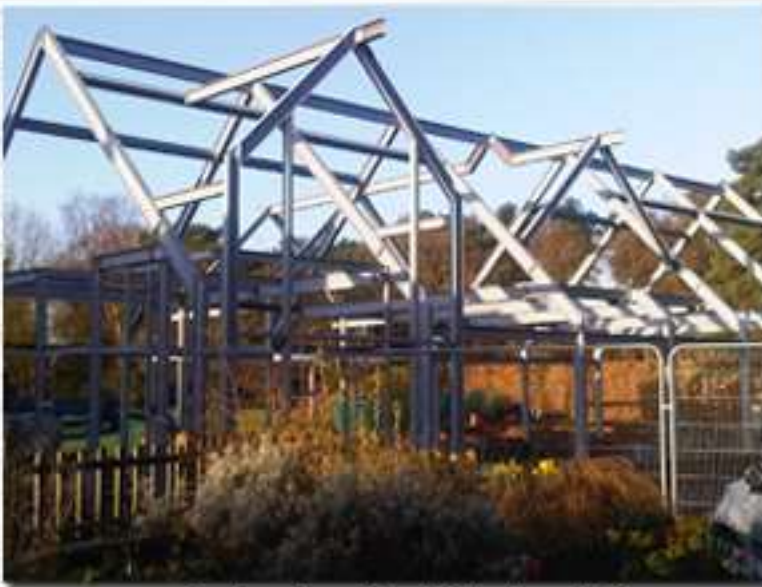
Swimming Pool Steelwork 3
