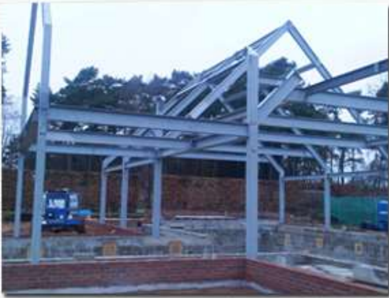
Swimming Pool Steelwork
