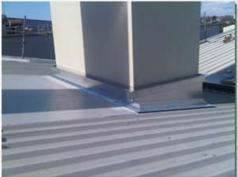
Flashing Ducts
