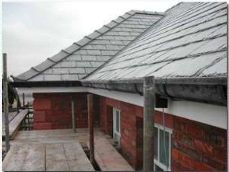
Fitting aluminum cast gutters
