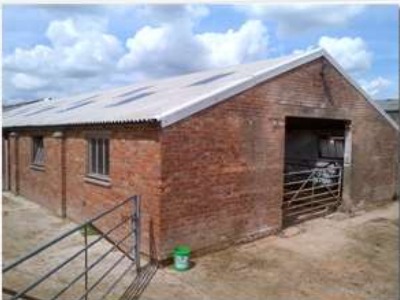
Re-roof, gutters and raised door height
