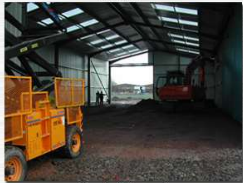
New build internal
