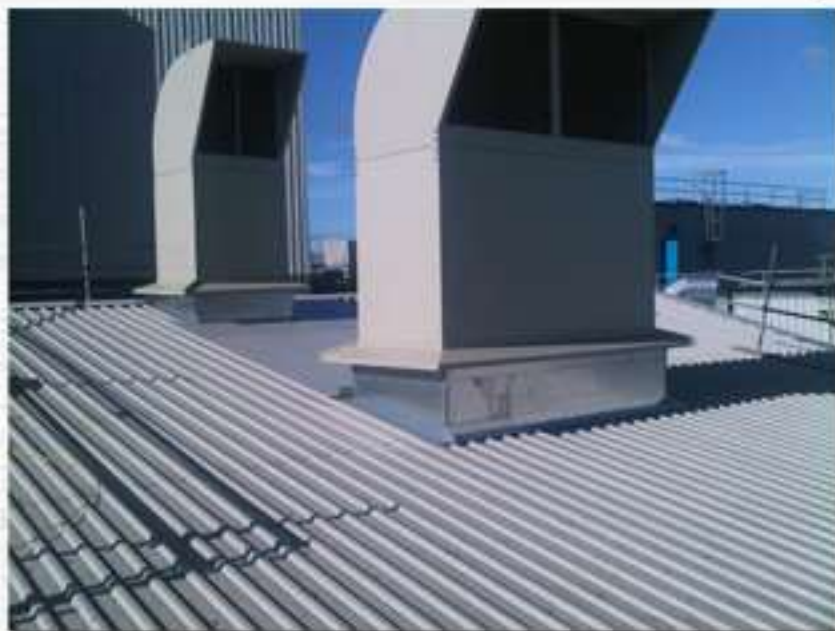
Fitting Flashings Around Installations
