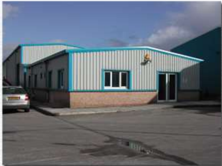
Install new windows & flashings
