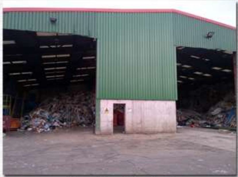
Recycle Plant Repairs 2
