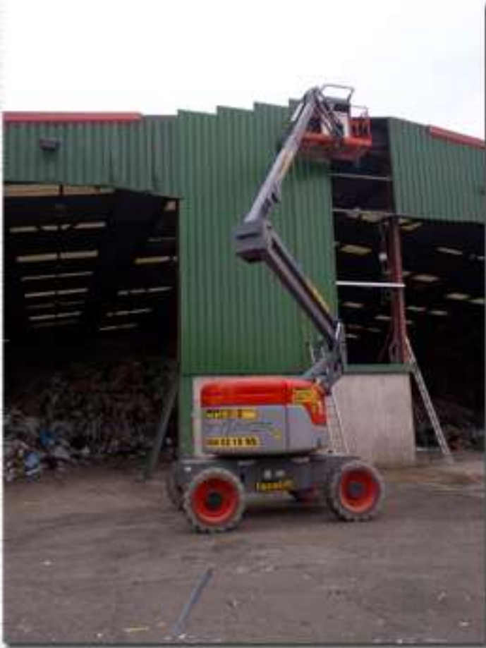
Recycle Plant Repairs
